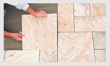
Sand and cement render - Natural stone tiles can be fixed directly onto sand and cement renders, they make an ideal surface for a successful installation. Sound render has a maximum loading bearing capacity of 40KG per sqm. All render must be fully dry before commencing installation, you must allow at least two weeks for internal applications and three weeks for external. The moisture level must be checked before commencing work as climatic conditions can vary drying times.
