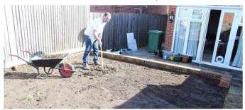
Once this has been completed its time to compact the base material, the best option is to hire a plate compactor as shown below. Compact the whole area a number of times, with each time you might need to do a little more levelling as the base material will not always compact evenly. Don't forget that the level of your base should be around 10-20mm below your lawn edgings to allow for your chosen Authentic Lawns product to finish at the right height.
