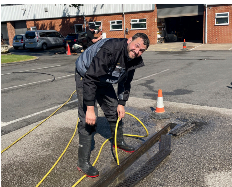
Pete helps the maintenance team with problem drains.
